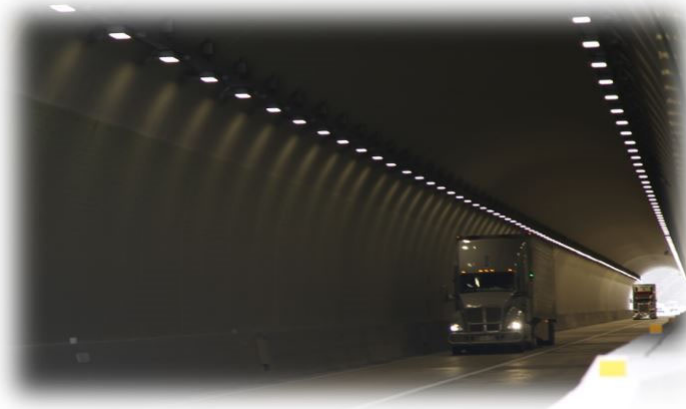
Figure 27: LED Lighting in the Carlin, Nevada Tunnel
