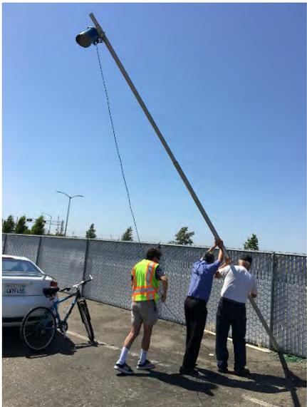
*Pole was lowered and mounting height of radar detector raised to 20 feet*
